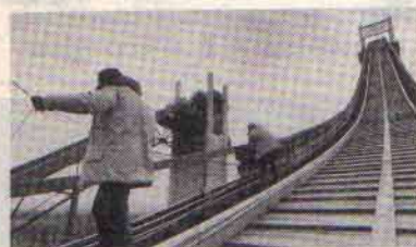
Ski jumping coverage was coordinated by two mobile vans parked under 70-meter jumping tower. Both 70- and 90-meter towers were completely rewired shortly following the construction of the towers themselves
