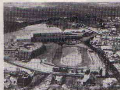
Coverage of skating events was coordinated through mobile vans parked behind new Olympic Center behind Lake Placid High School. Platforms on high school itself provided master shots of speed skating oval and Main Street
