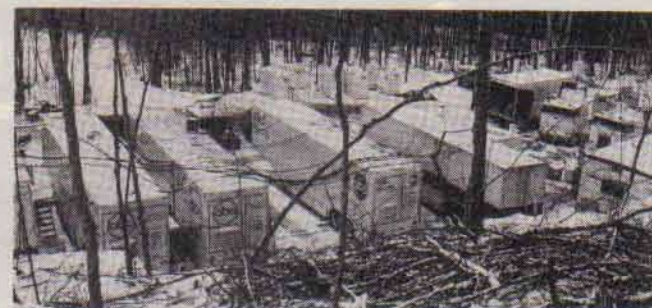
Whiteface Mountain was the venue for alpine skiing events, coordinated through a complex of mobile vans parked 1000 feet uphill from base lodge in a small clearing. Cameras on small wooden pallets could be transported from one slope to another by helicopter. For longer cable runs, special RF repeaters developed by Phillips for its LDK cameras, used extensively at the venue, provided triax runs up to 15,000 feet
